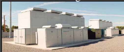
Energy Storage – MV and LV
