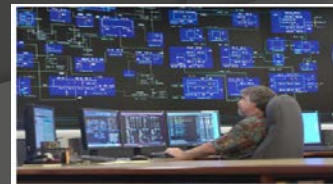
Grid Control Center
