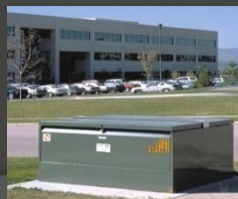
Pad Mounted Switches
