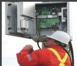
SCADA switches
